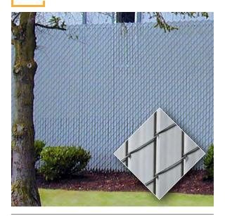
Industrial Pre-Woven is a standard styled slat that is mechanically inserted into the chain link wire fabric during the weaving process. Once inserted, the wire is finished above and below the slat (either bow-knuckle or knuckle-over).
