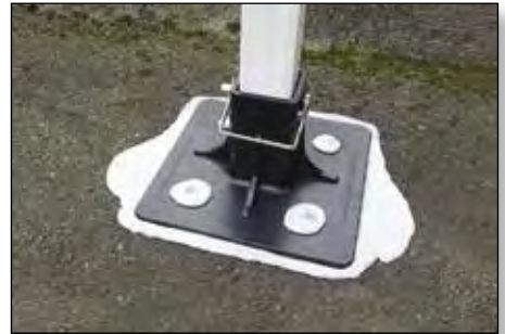
Quick Release Pin base installed with epoxy
