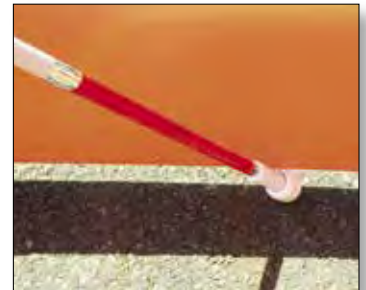
The bottom panel acts as a detectable edge for pedestrians using canes
