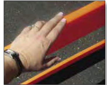
The top panel acts as a smooth continuous guide for the hand
